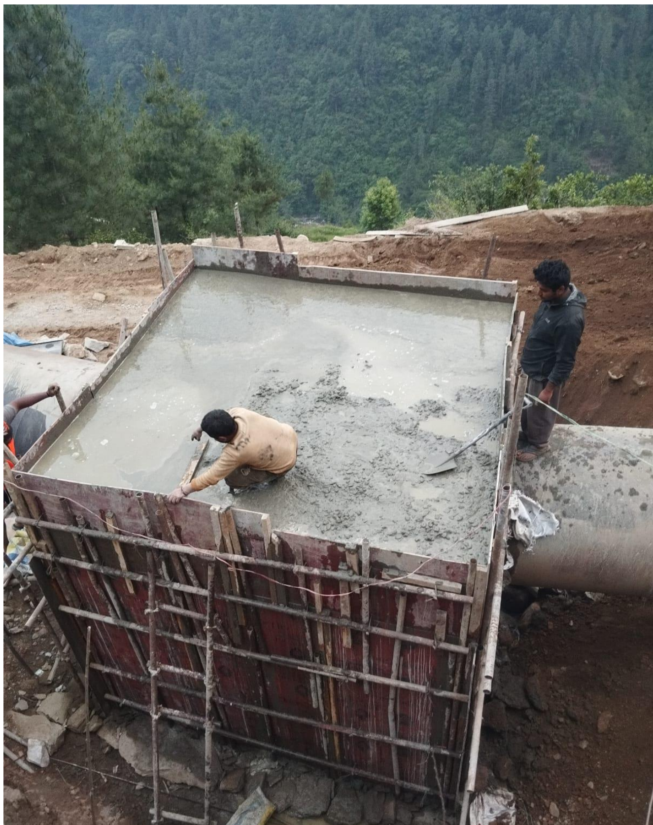
Figure 8: Ongoing concrete work at anchor block 35, final level touch up.
