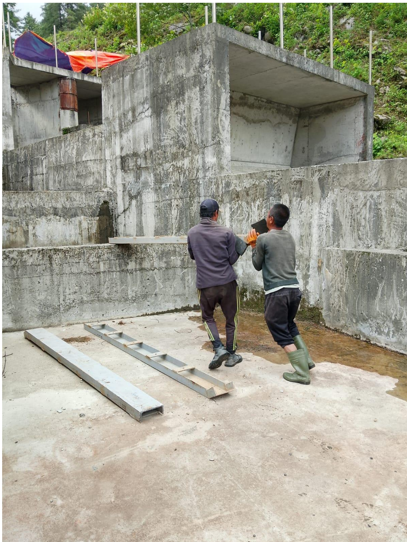
Figure 13:HM work progress ongoing Gravel flushing Gate frame installation work at site.
