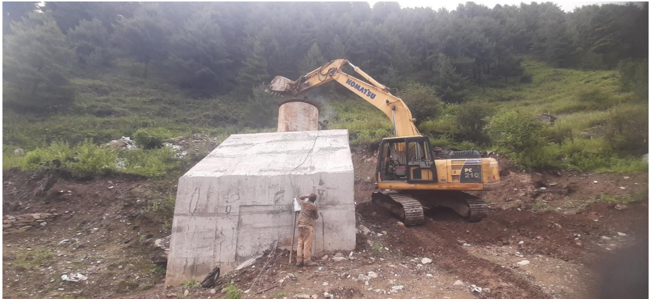
Figure 16: HM work progress at site, installation of ms cover at the top of the surge pipe with the provision of air release.
