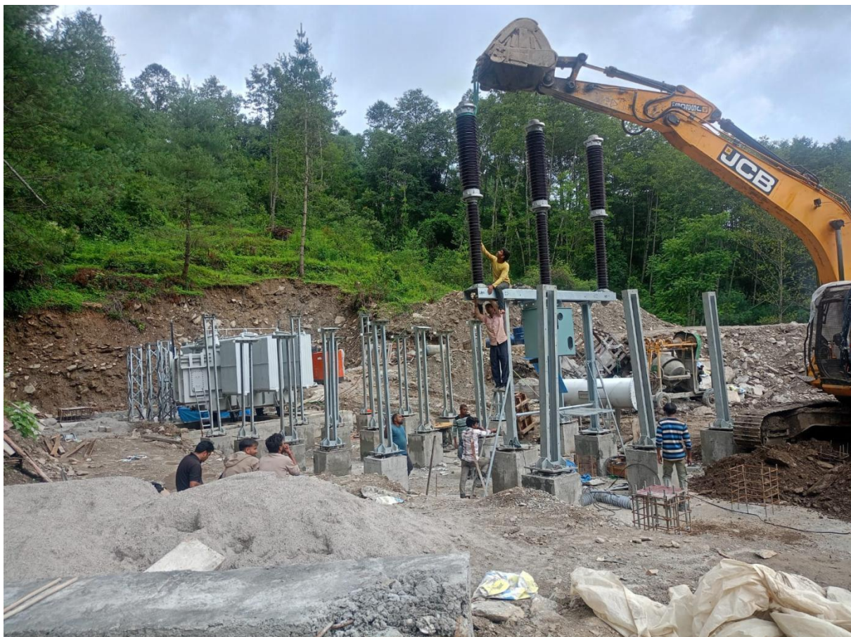
Figure 29: Installation of 132 kV breaker bushing completed
