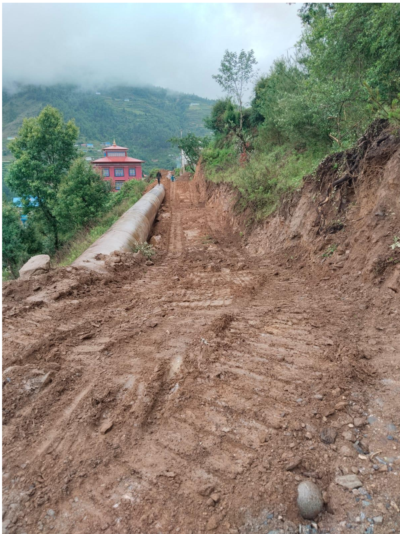
Figure 7: Work progress along headrace pipe alignment, ongoing road and alignment excavation.
