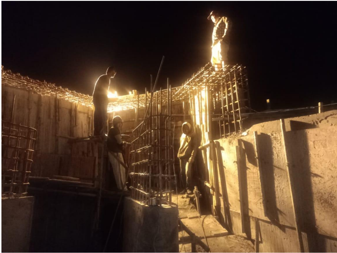
Figure 4: Late Night work at settling basin conveyance tank area, ongoing rebar work.
