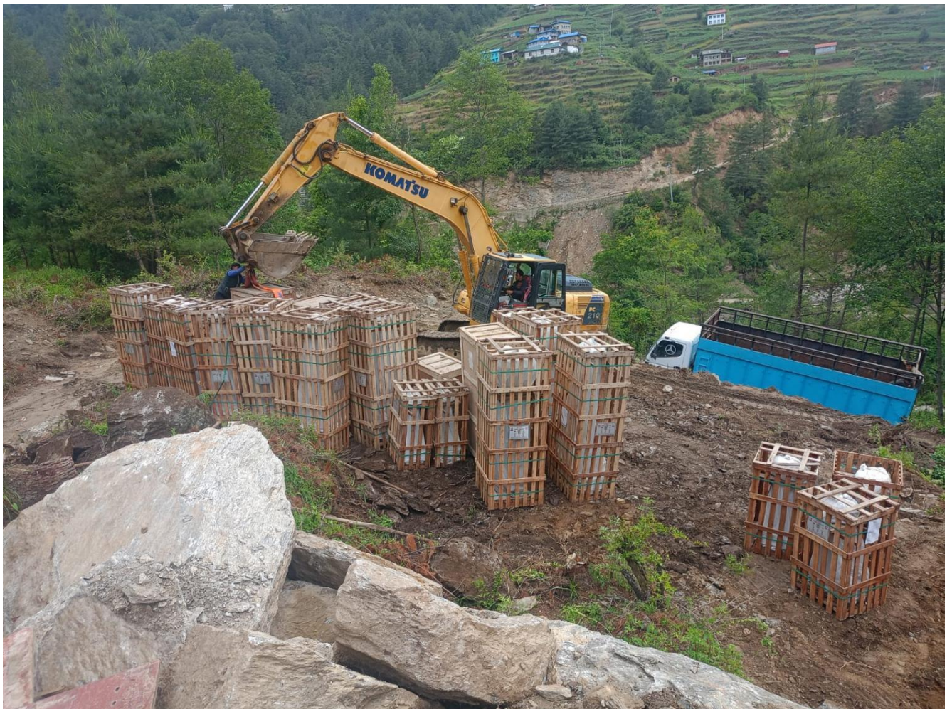
Figure 27: Interconnecting substation equipment transported and stored at site.
