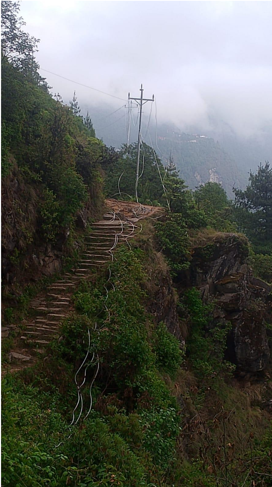
Figure 24: Conductor spreading and laying on the ground for straining.
