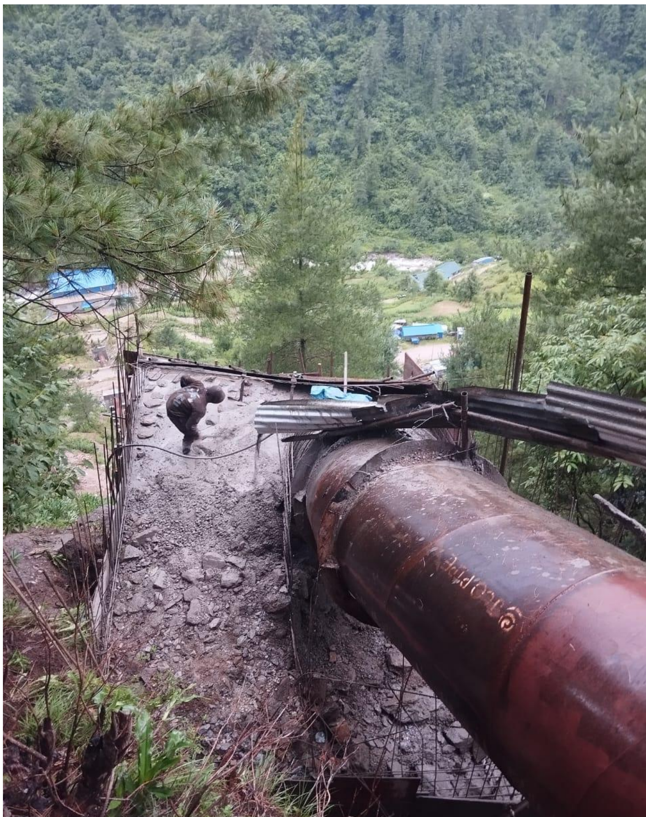
Figure 11: A view of penstock alignment, ongoing concrete work at penstock anchor block PVB-03.
