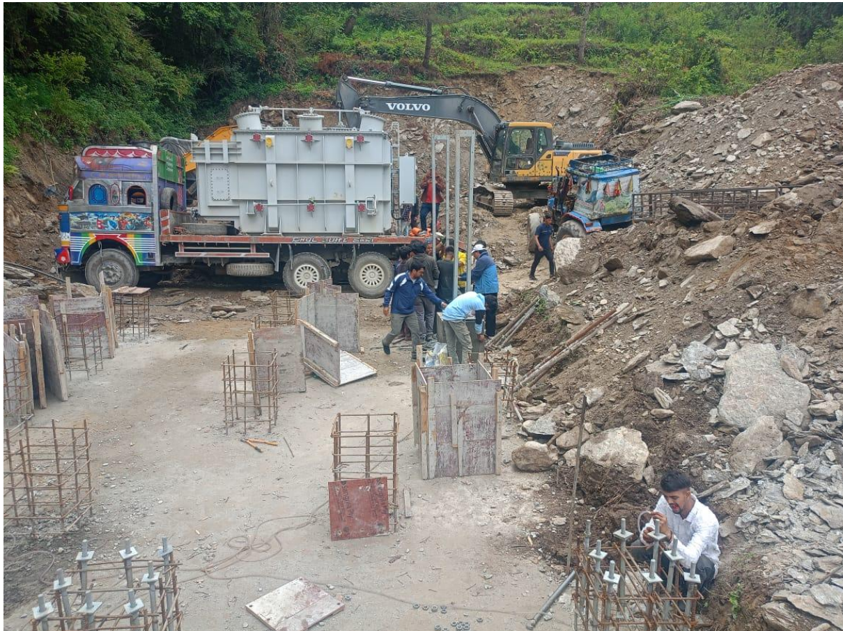
Figure 28: Transformer shifted from the yard to the transformer foundation.
