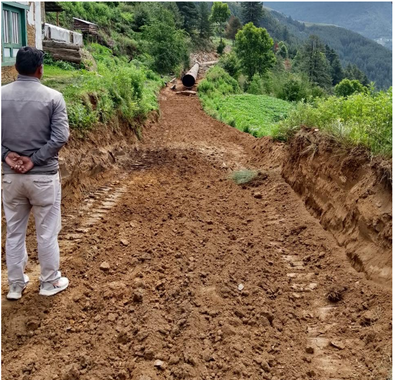
Figure 6: Work progress along headrace pipe alignment, excavation for pipe erection at ch 2+750.
