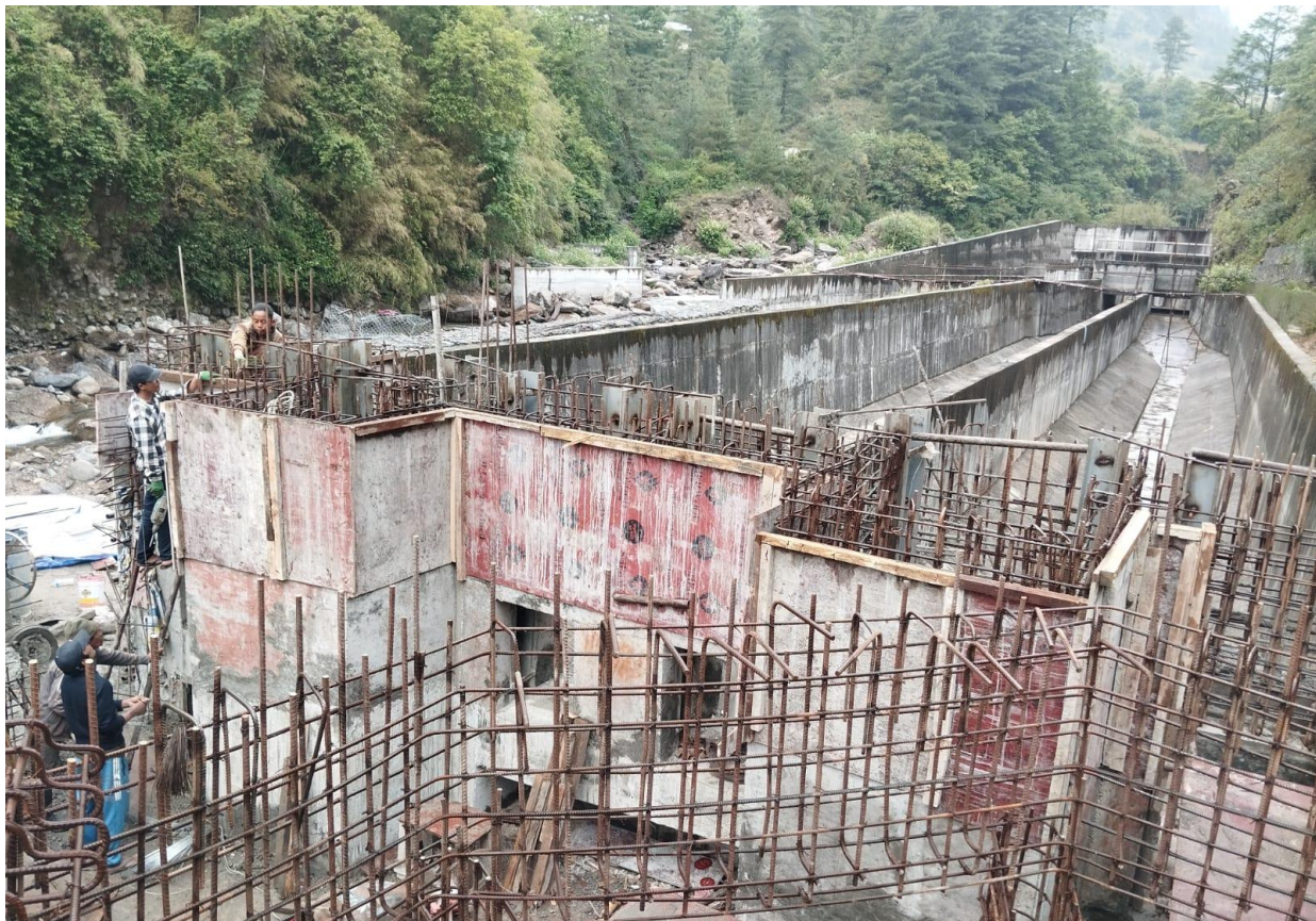
Figure 3: A close view of settling basin, conveyance tank, ongoing rebar and formwork.
