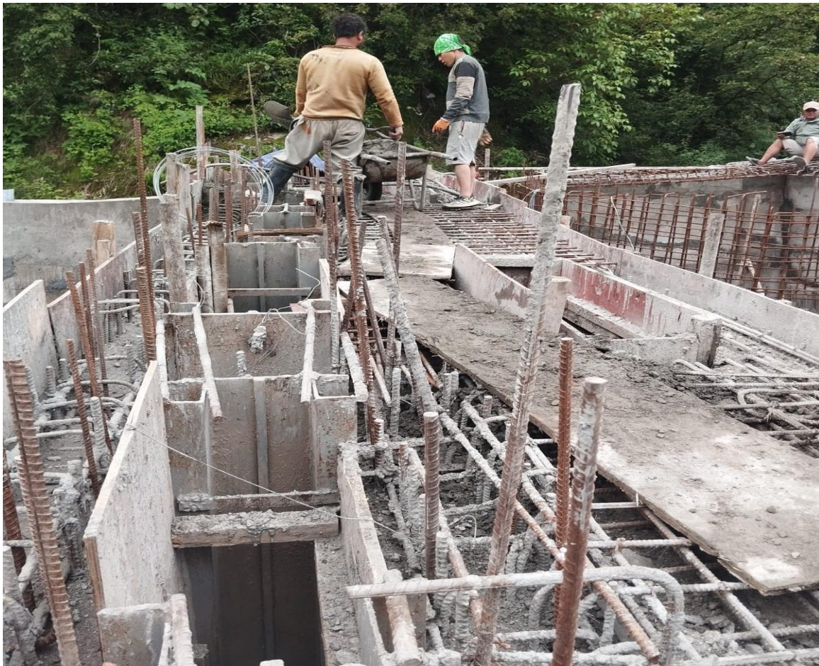
Figure 5: Ongoing concrete work at the top slab of settling basin outlet.
