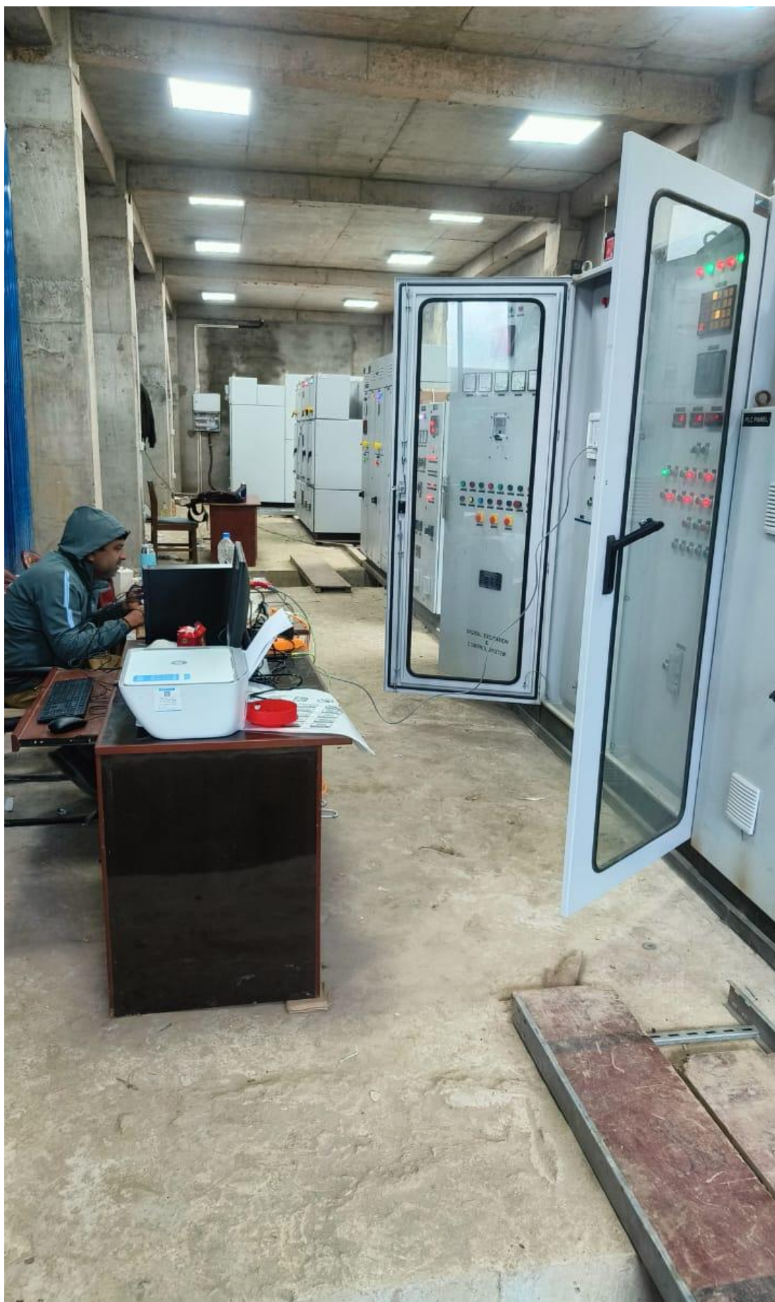
Figure 21: Ongoing EM work inside the powerhouse, checking of panels in control building.
