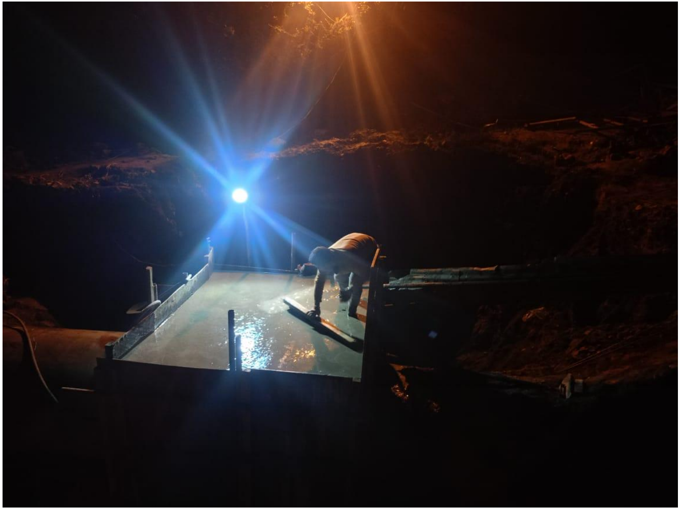
Figure 9: Ongoing late night work, completion of concrete work at anchor block 36'.
