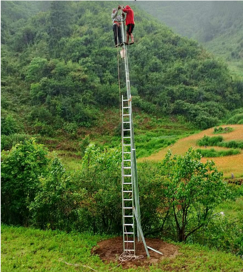
Figure 22: Channel fixing work in single pole 33kV Transmission Line.
