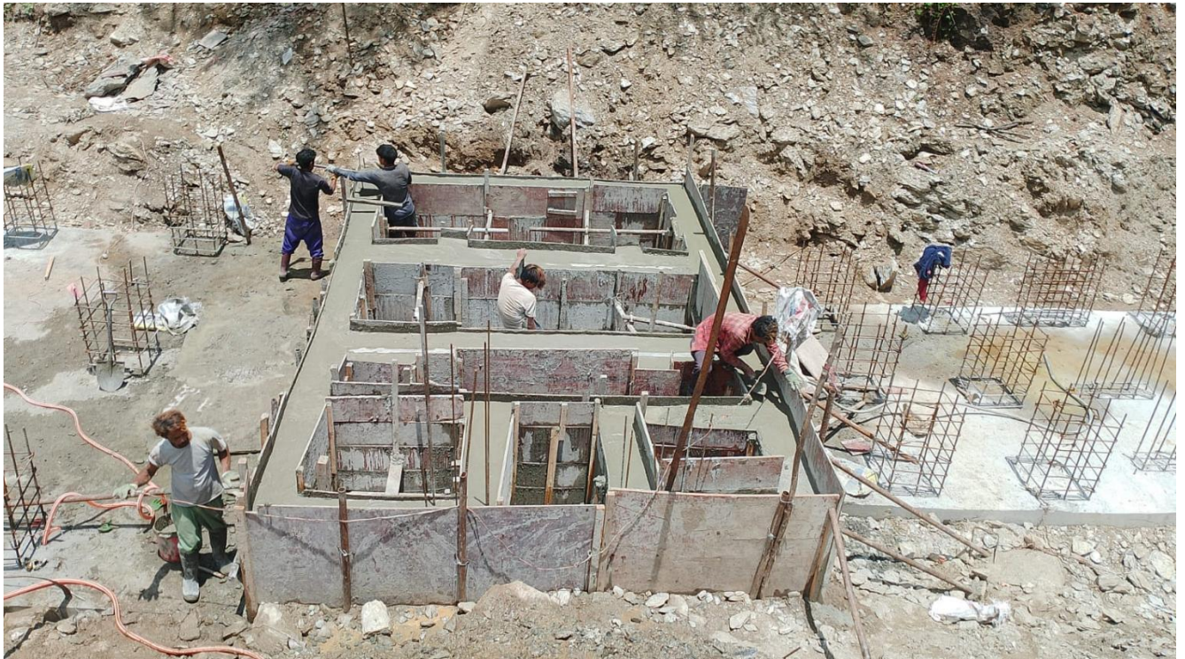
Figure 26: Power transformer (33/132 kV) foundation construction completed.
