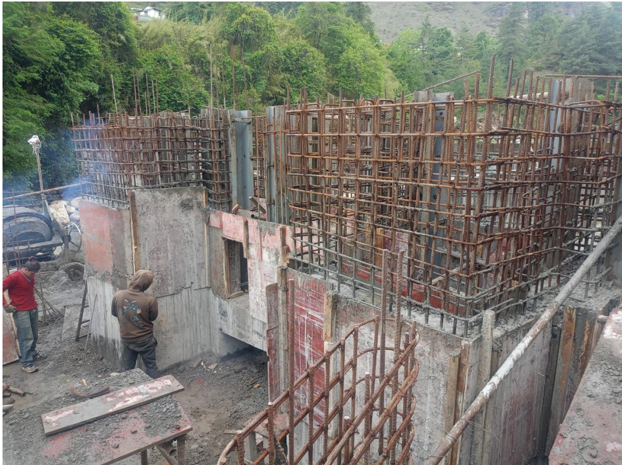
Figure 2:Ongoing Rebar binding and formwork fixing in settling basin conveyance tank area.
