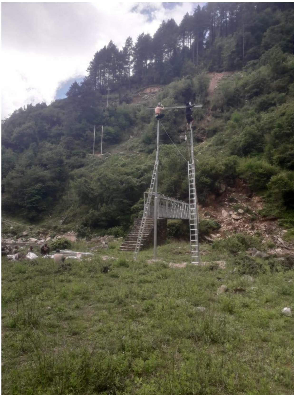
Figure 23: Arm channel fitting work in Transmission line alignment.
