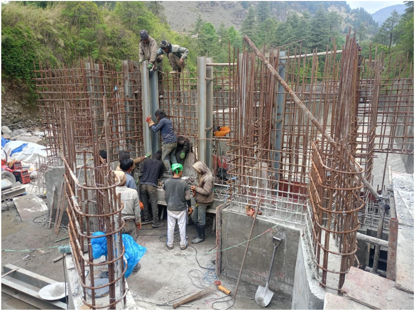
Figure 14: HM work progress at site, Installation of settling basin outlet gate frame, viewing U/S.
