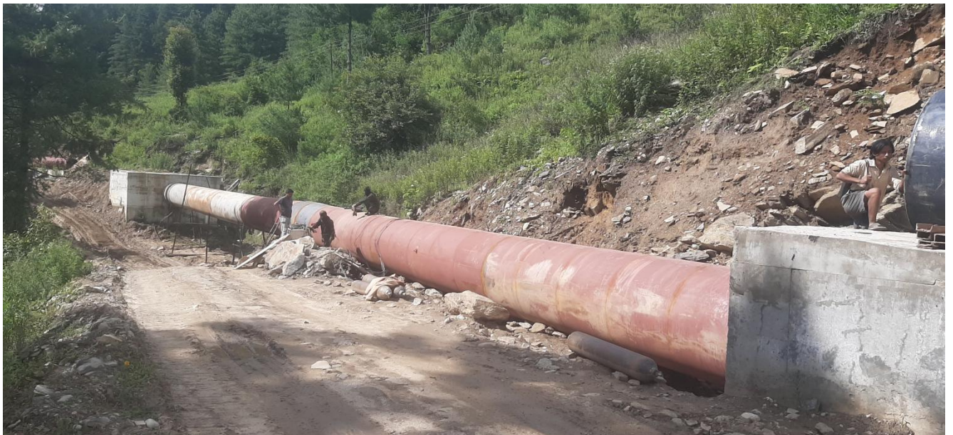
Figure 15: HM work progress at site, Headrace pipe erection work complete, viewing U/S from chainage 1+780.
