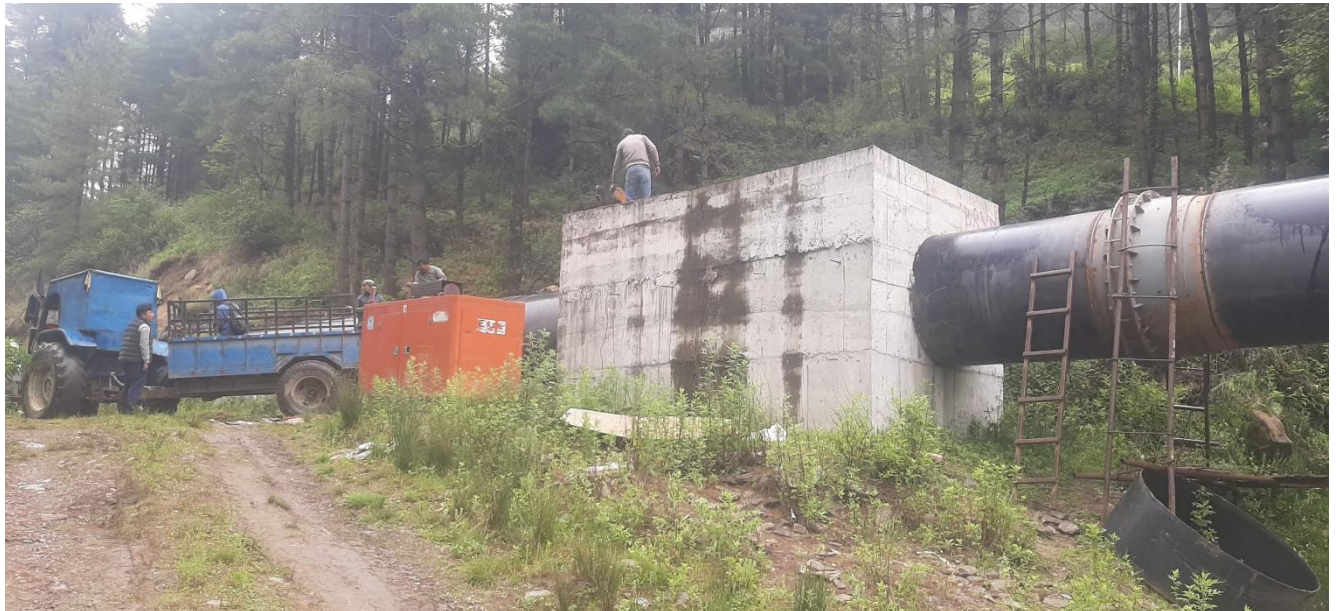
Figure 17: HM work progress at site, ongoing erection of expansion joint D/S of anchor block 16 along HRP.
